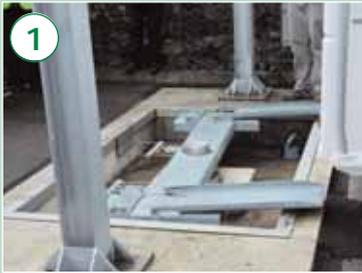
1. A carefully-balanced cross-beam has a central pivot; springs keep it centrally aligned at rest
